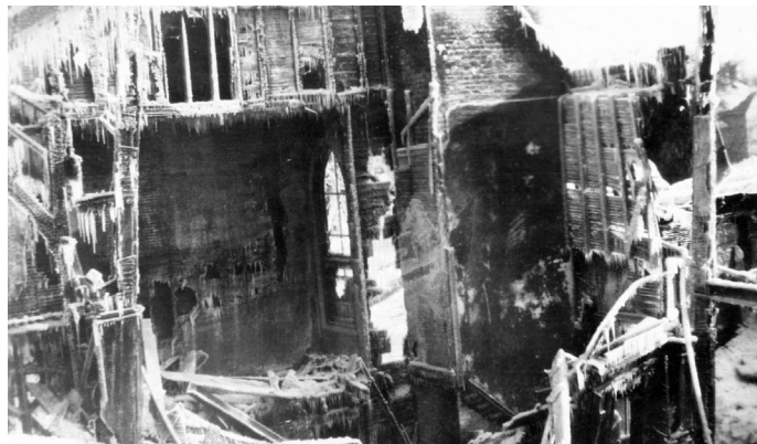
Interior after fire
